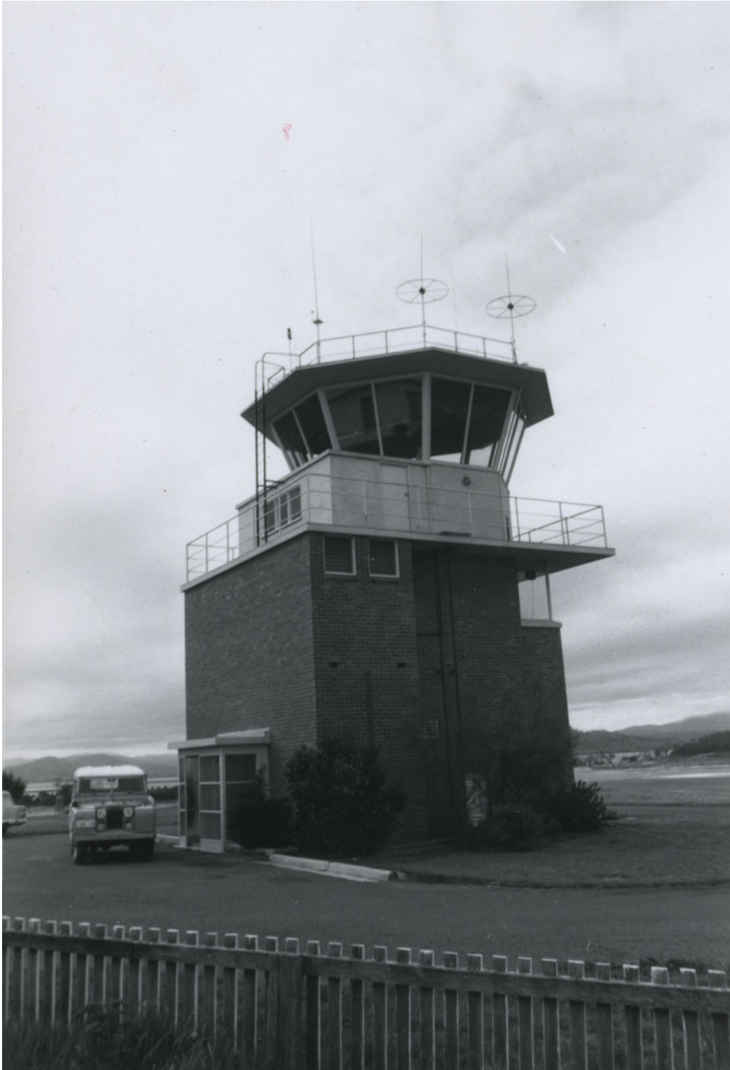
Figure 18 Undated, c. 1970s, view of the ATC tower looking north-west: note the original entry enclosure:
