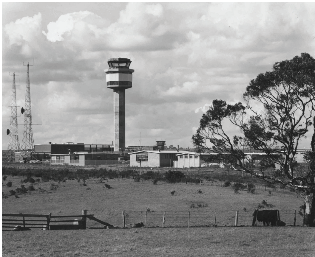
Figure 54 View of the Tullamarine ATC tower, c. late-1960s
