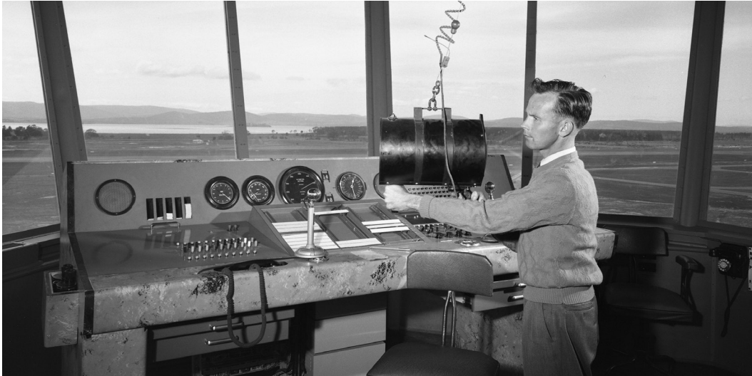
Figure 16 Hobart control tower cabin, 1958, with the hand-held, roof mounted beacon on display
