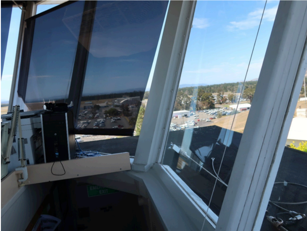
Figure 45 The canted steel-framed windows are original
