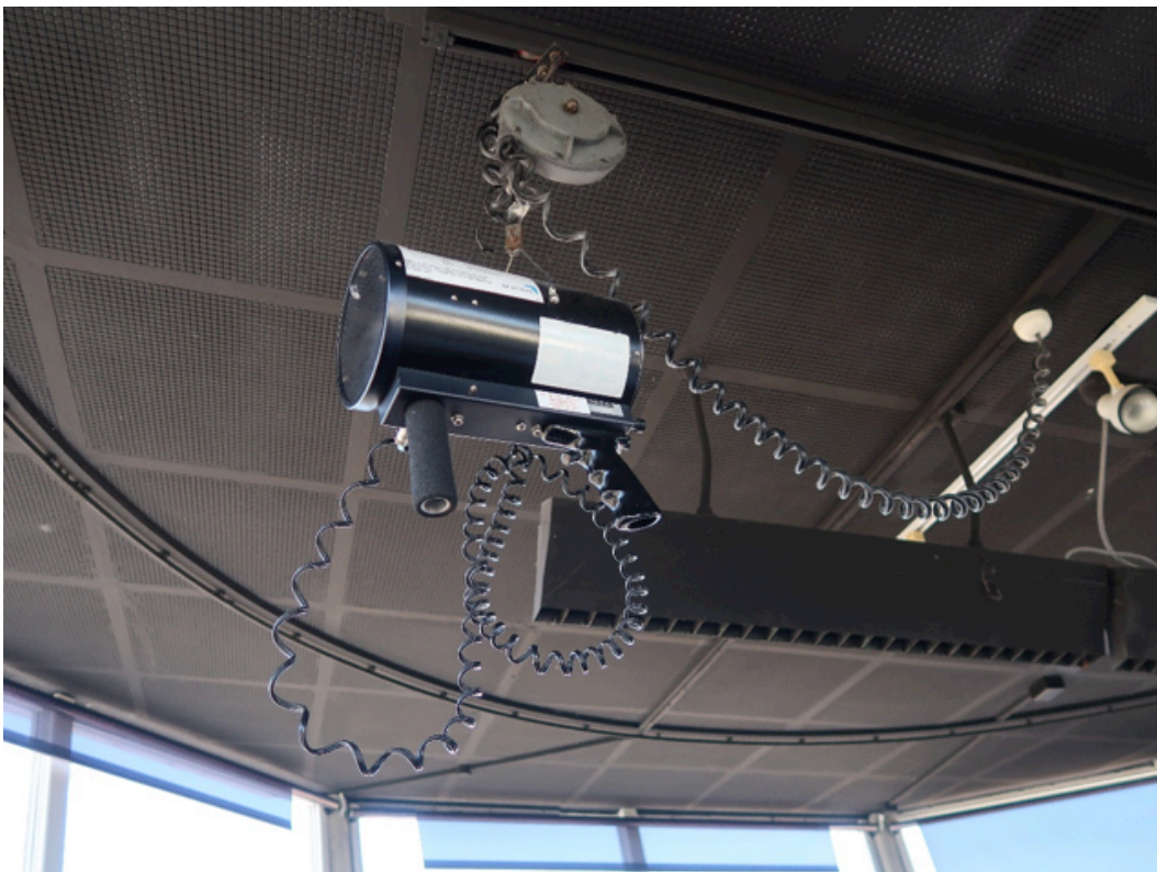
Figure 46 The perforated acoustic tiles, 'egg crate light', hand-held beacon and the circular visor track are original
