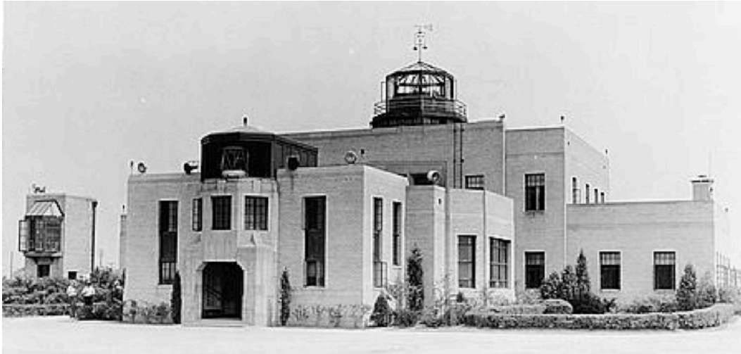
Figure 51 Airport building with roof-mounted air traffic control cabin at Cleveland Airport, Ohio, USA, 1929
