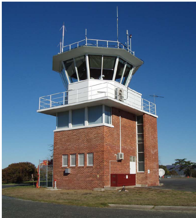
Above: North and east elevations of Hobart Control Tower. The exterior is essentially intact as completed in 1958
