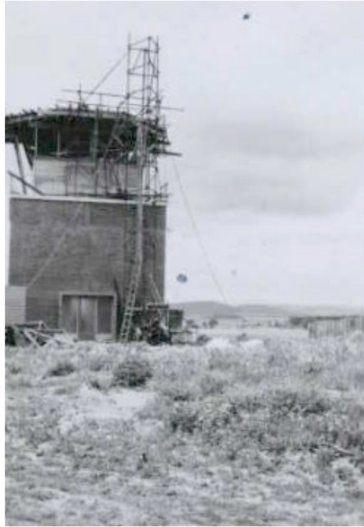
Figure 13 Left and right: Hobart ATC tower under construction, 30 November 1956: west and north elevations (left) and south elevation (right)
