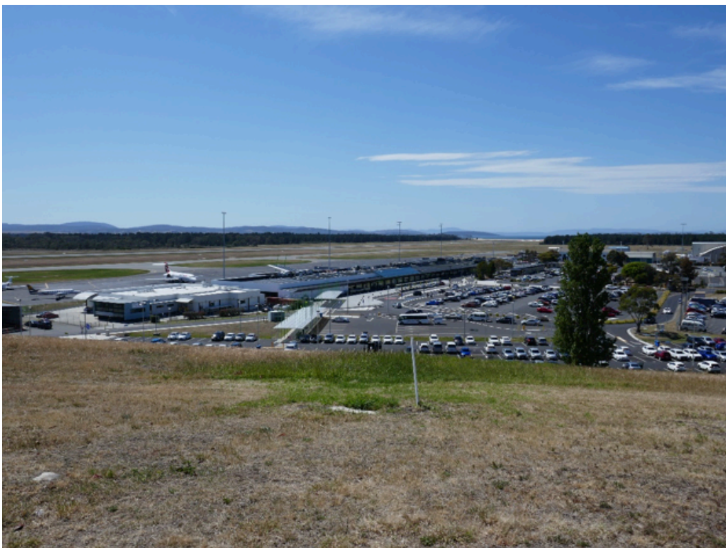
Figure 49 View looking south-east from the base of the ATC tower
