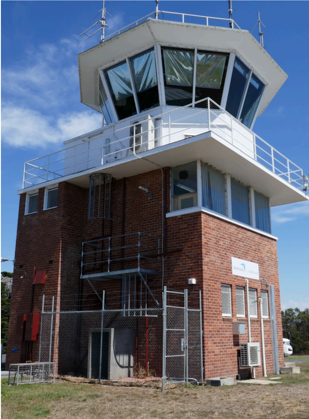
Figure 28 East (left) and north, part (right) elevations of the ATC tower
