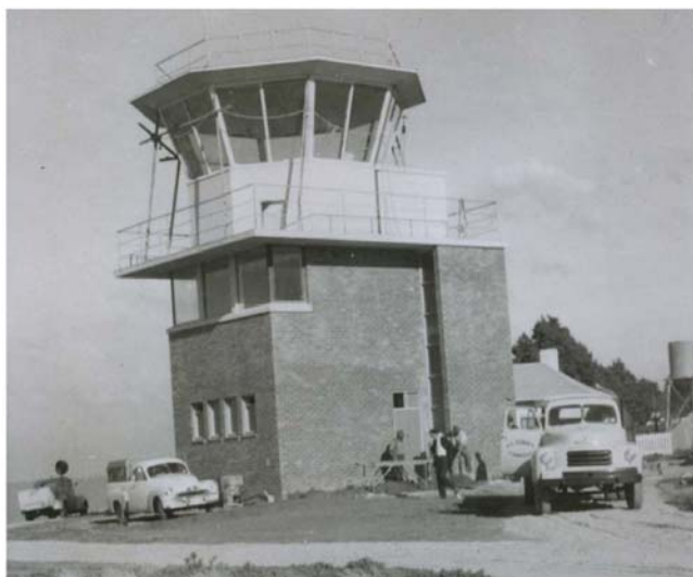
Above: View of tower during construction May 1957
