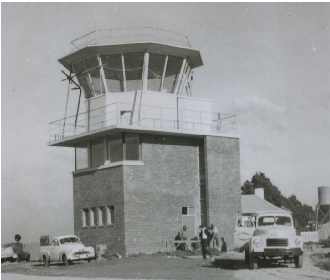
Figure 14 Hobart ATC tower under construction, 7 May 1957: north and west elevations
