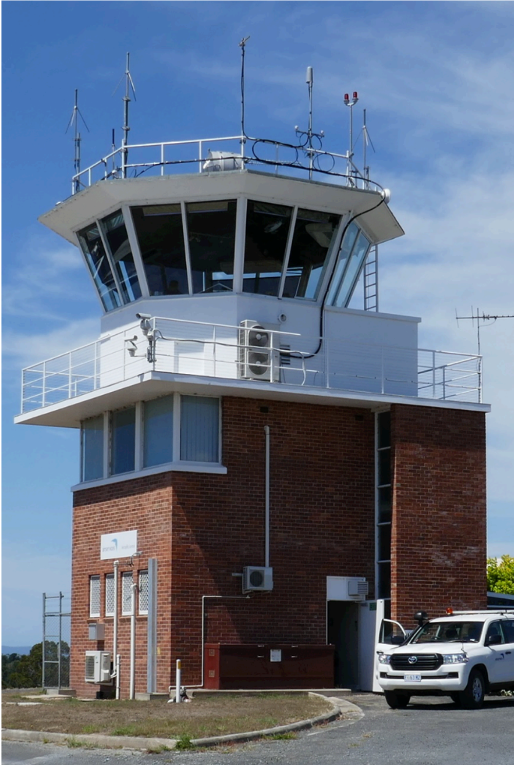
Figure 31 West elevation: note double-height casement window to the north-facing elevation of the stairwell (pictured right)
