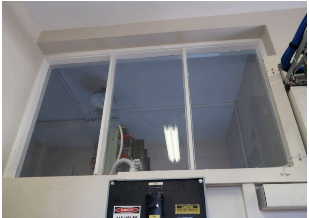
Figure 35 Highlight window between the equipment and switch rooms
