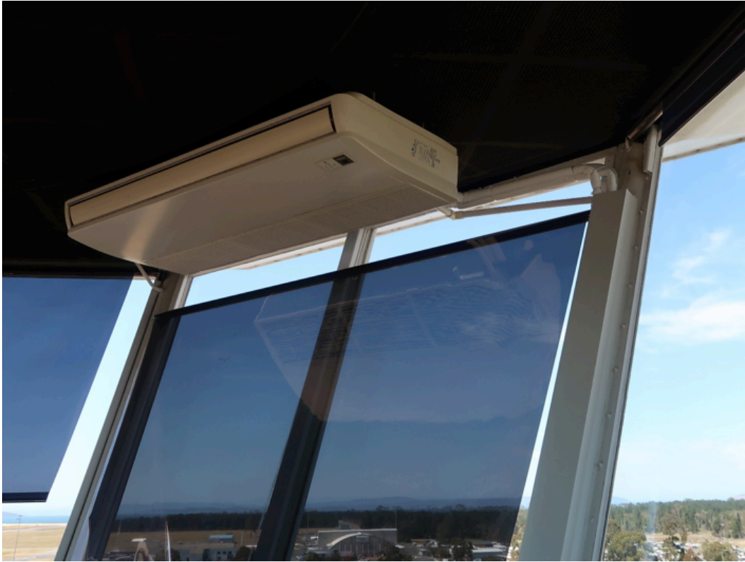
Figure 55 Hobart ATC tower cabin: note the thick mullions and frames
