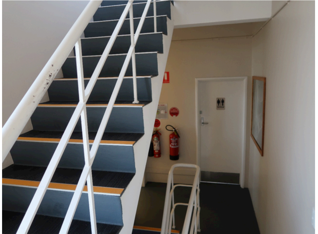
Figure 38 First floor: view looking east from the staircase
