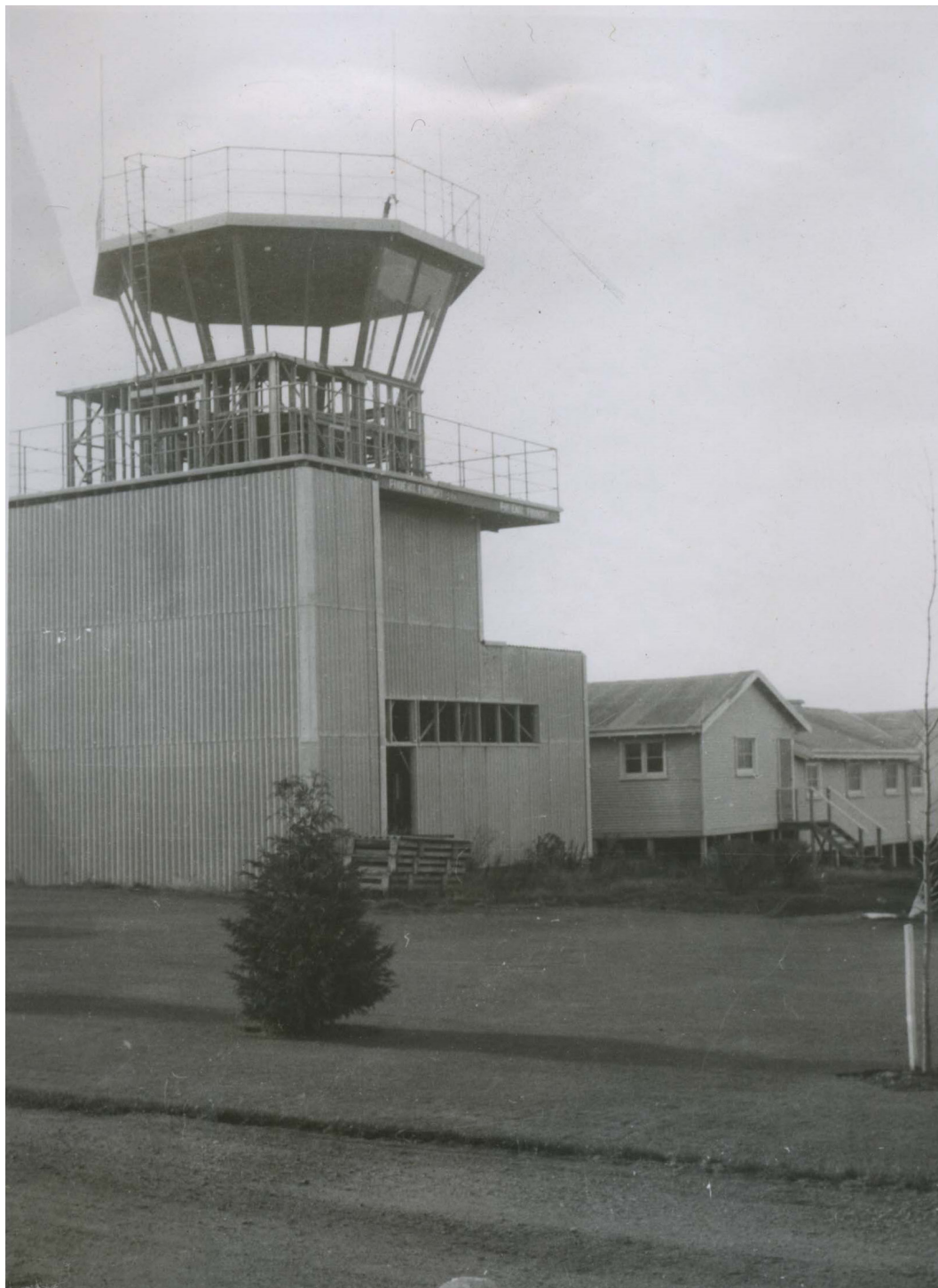
Figure 12 Launceston ATC tower under construction, 9 May 1957: the Air Traffic Control Centre to the right of picture was a former 7EFTS building
