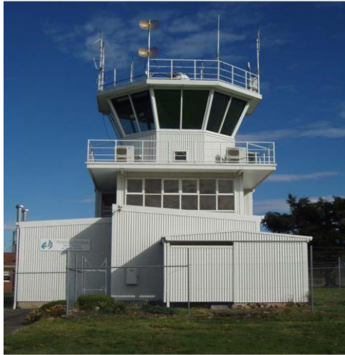
Above: North-east elevation, 2008. Note 1960s extension to equipment room (left)
