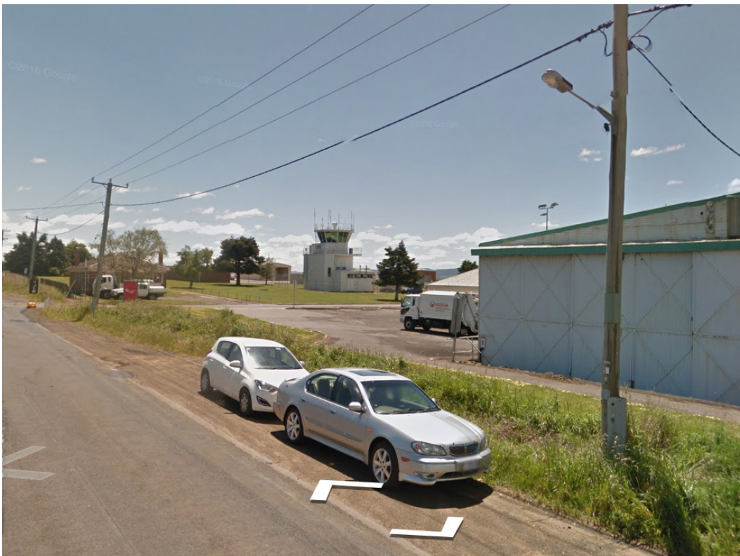
Figure 42 View looking north-west along Evandale Road: the ATC tower is visible in the centre
