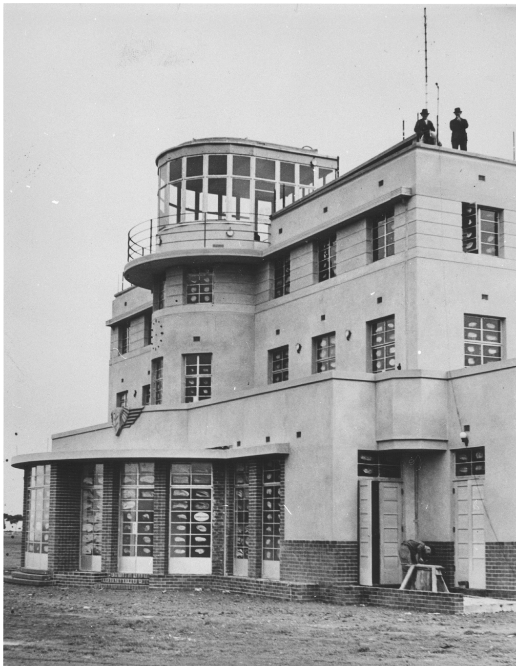
Figure 45 Airside elevation of Parafield (Adelaide) Operations and Administration Building, 1940, during construction
