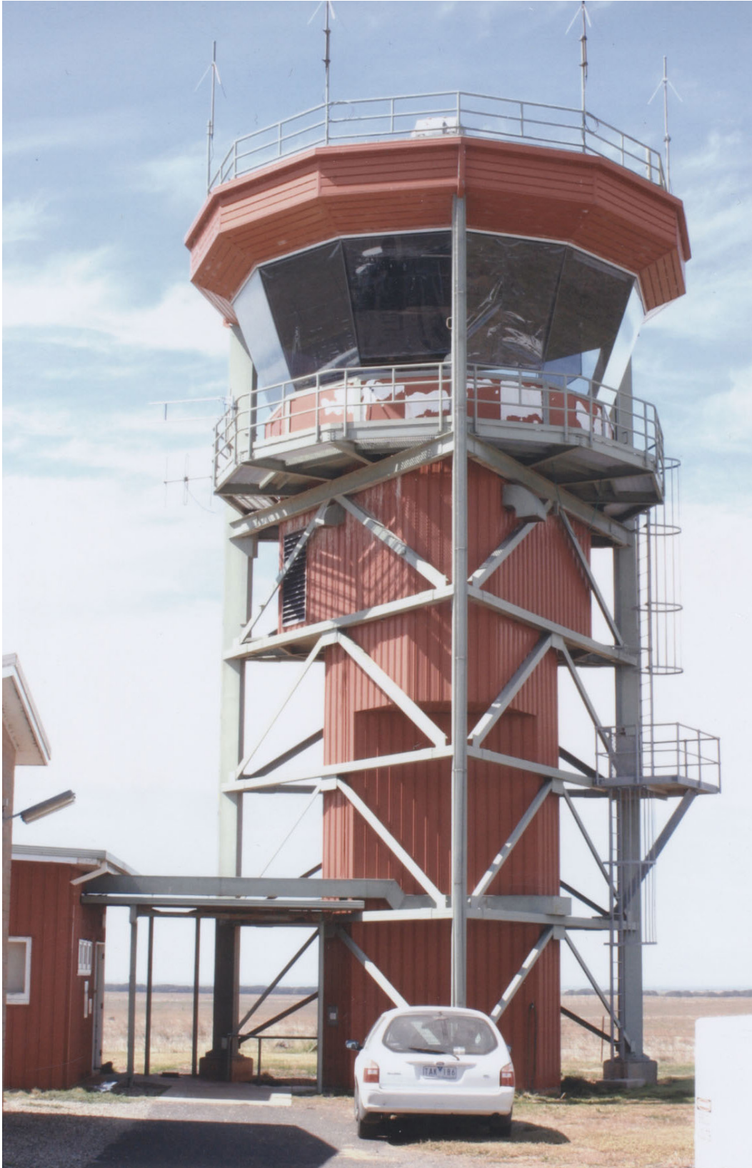
Figure 47 ATC tower at Avalon Airport, Victoria, 1980s
