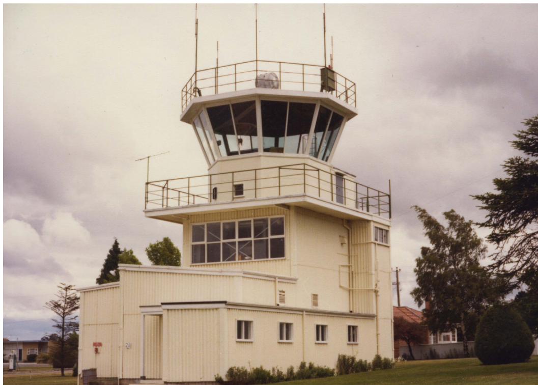
Figure 15 Launceston ATC tower, late-1970s, north-east and north-west elevations: the skillion-roofed enclosed corridor in the foreground is a remnant of the link to the Control Centre
