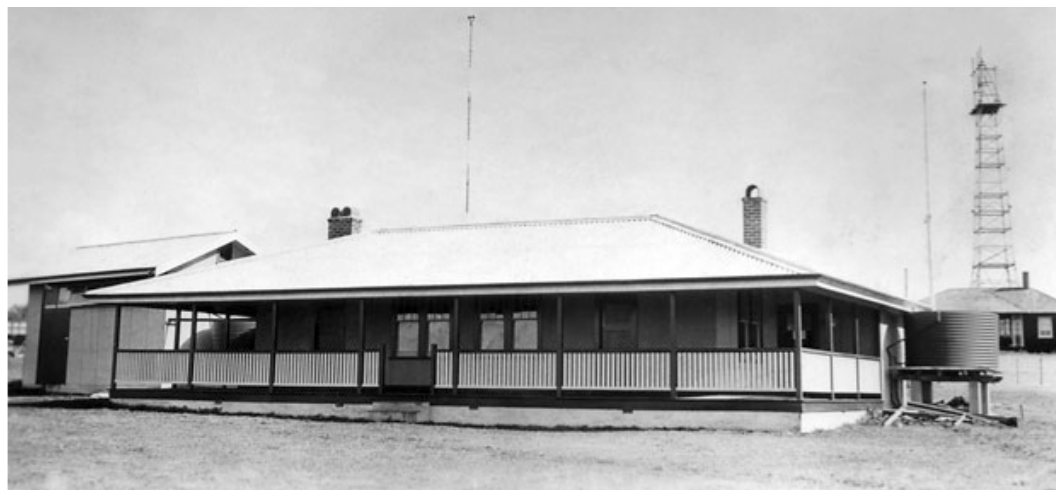
Figure 7 Launceston Aeradio station viewed from airside: the tall mast at right is a Lorenz 33 MHz Radio Range
