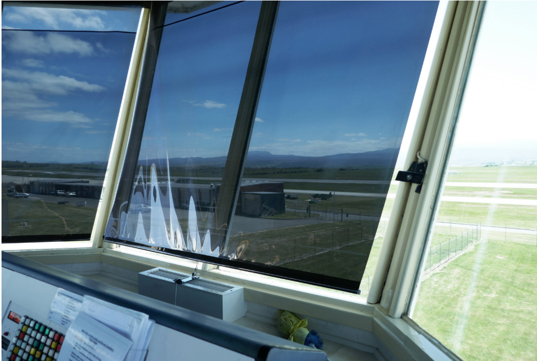
Figure 49 Launceston ATC tower no. 2 cabin: note the thick mullions and frames
