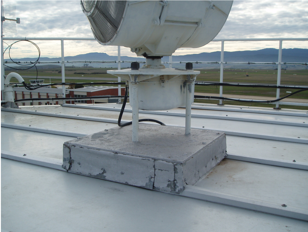
Figure 28 The roof of the ATC cabin (pictured in 2009)
