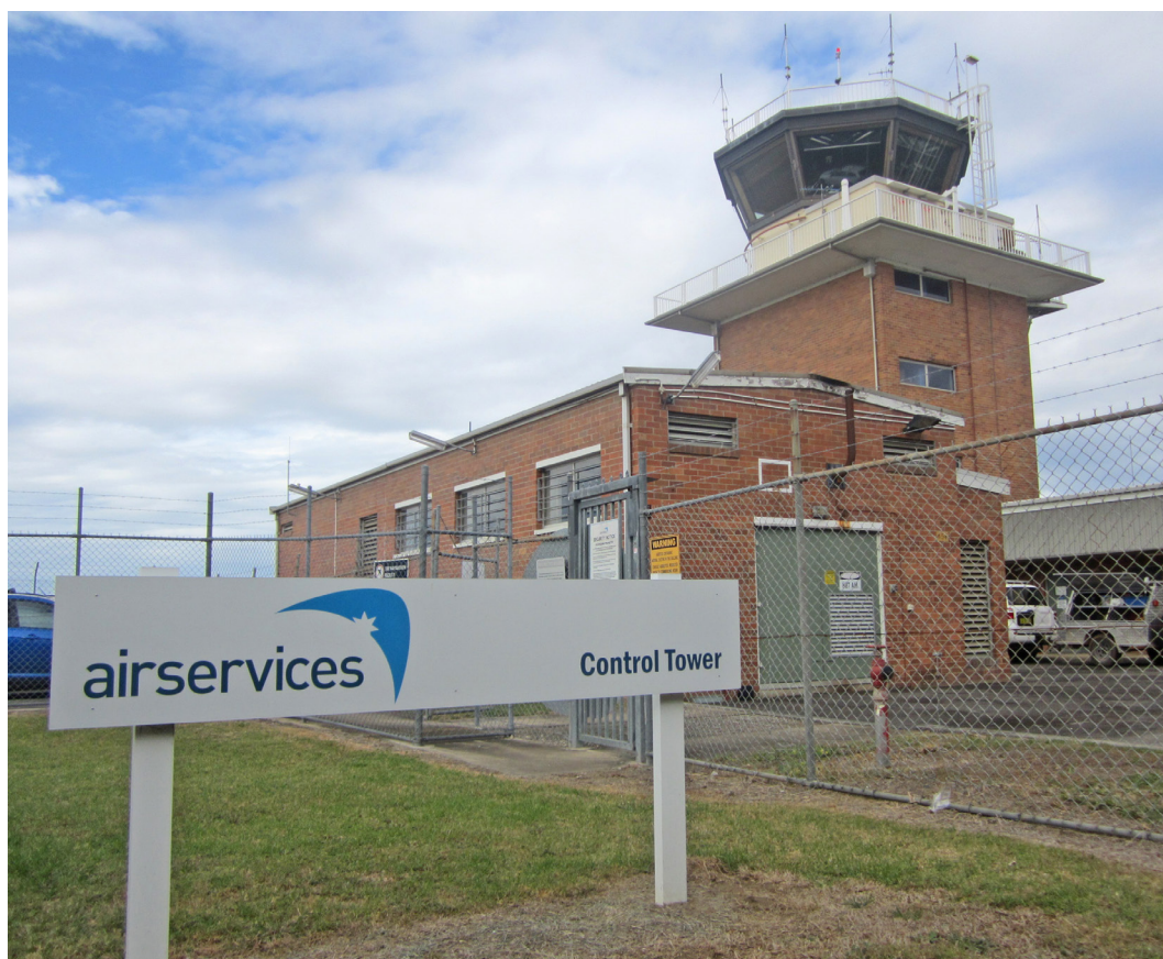
Figure 15 View of the Airservices compound at Bankstown from Tower Road, looking south-east: the power house is in the foreground and the radio equipment room is visible to the right
