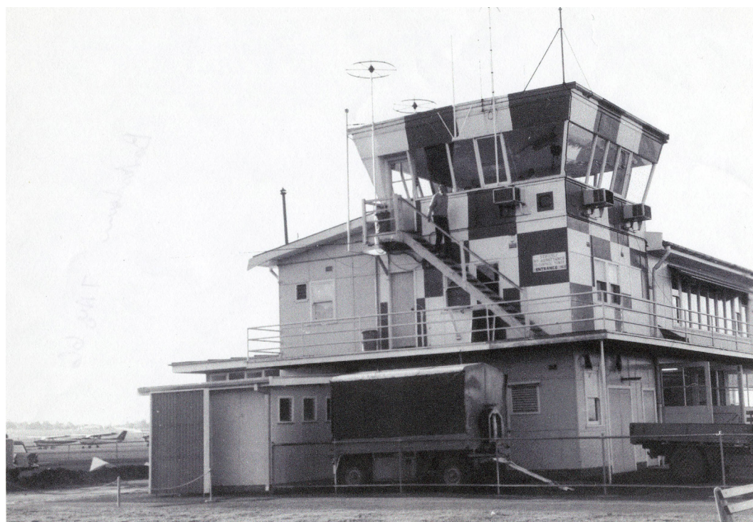
Figure 5 The RAAF tower at Bankstown (now demolished), 1966: view looking north-east
