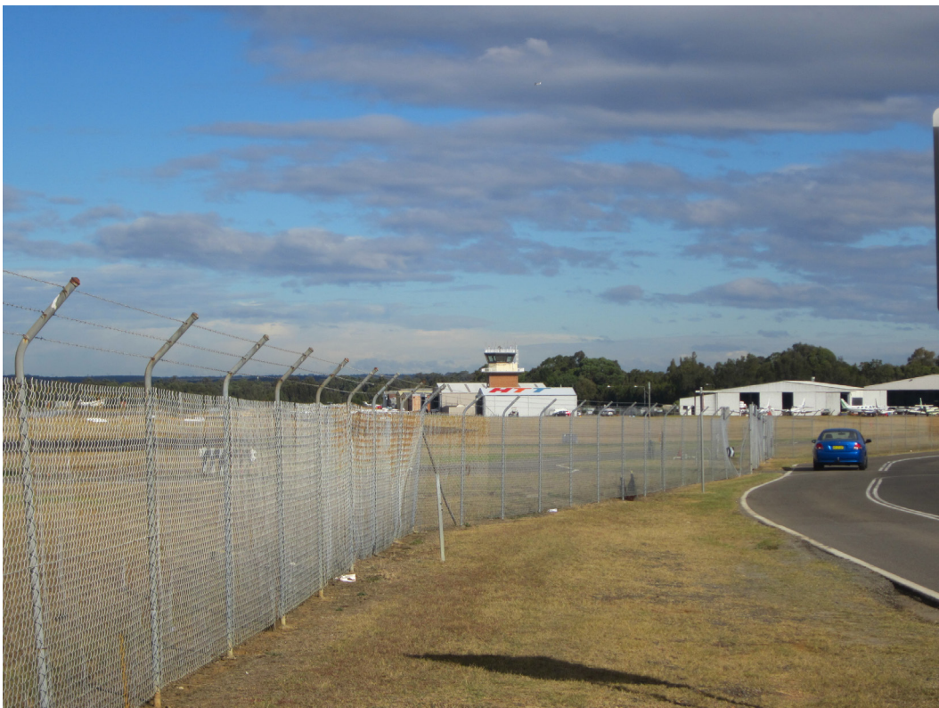
Figure 37 View looking south from Tower Road
