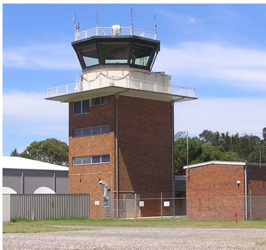
Above: East and north elevations, 2008. The powerhouse is to the right.
