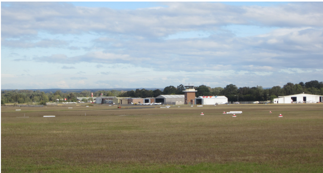
Figure 36 View of the Air Traffic Control tower from the north-east
