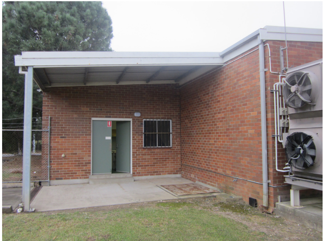
Figure 22 Radio equipment room: addition at the west end of the south elevation
