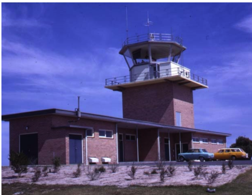
Figure 45 Jandakot ATC tower, Perth, (1965), integrated with single-storey equipment and service rooms
