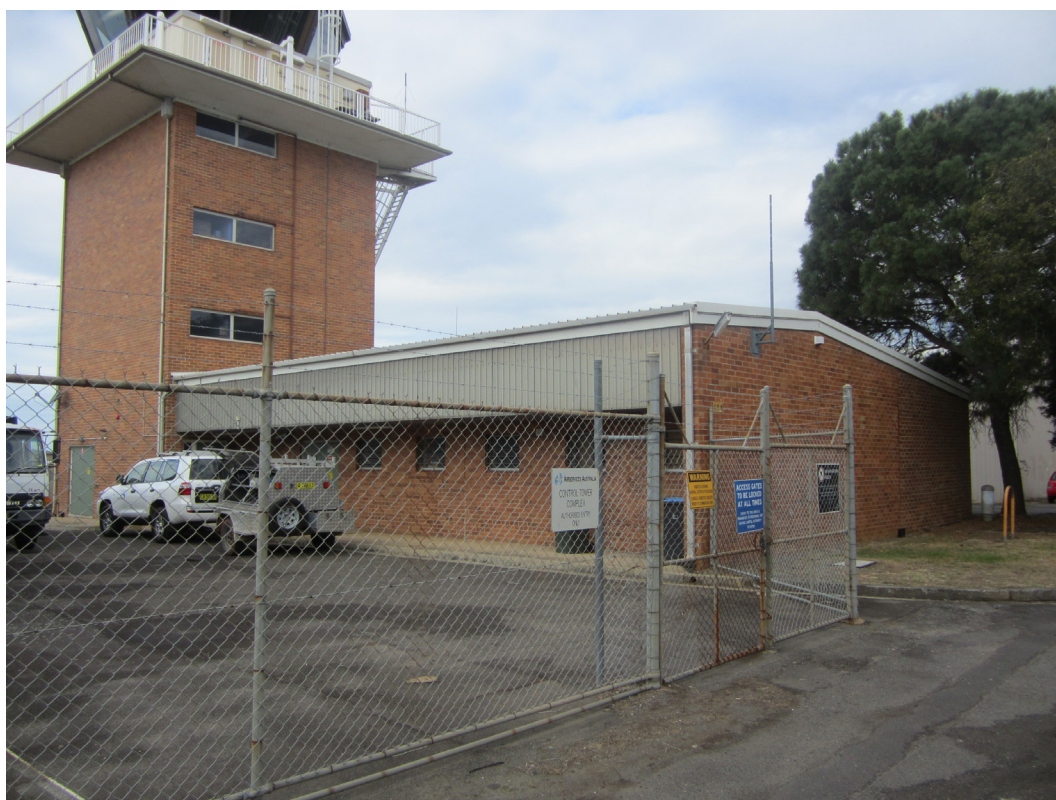
Figure 21 North and west elevations of the radio equipment room
