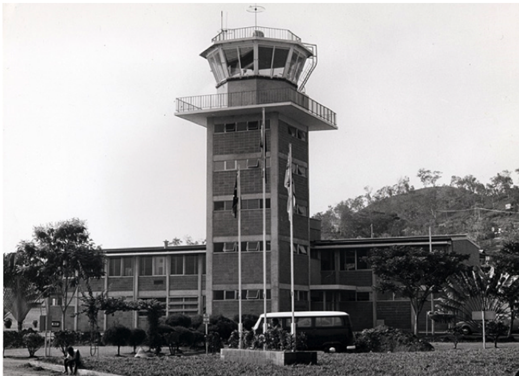
Figure 46 ATC tower at Port Moresby, Papua New Guinea, then an Australian mandated territory, early 1970s: a concrete-framed tower with brick panels
