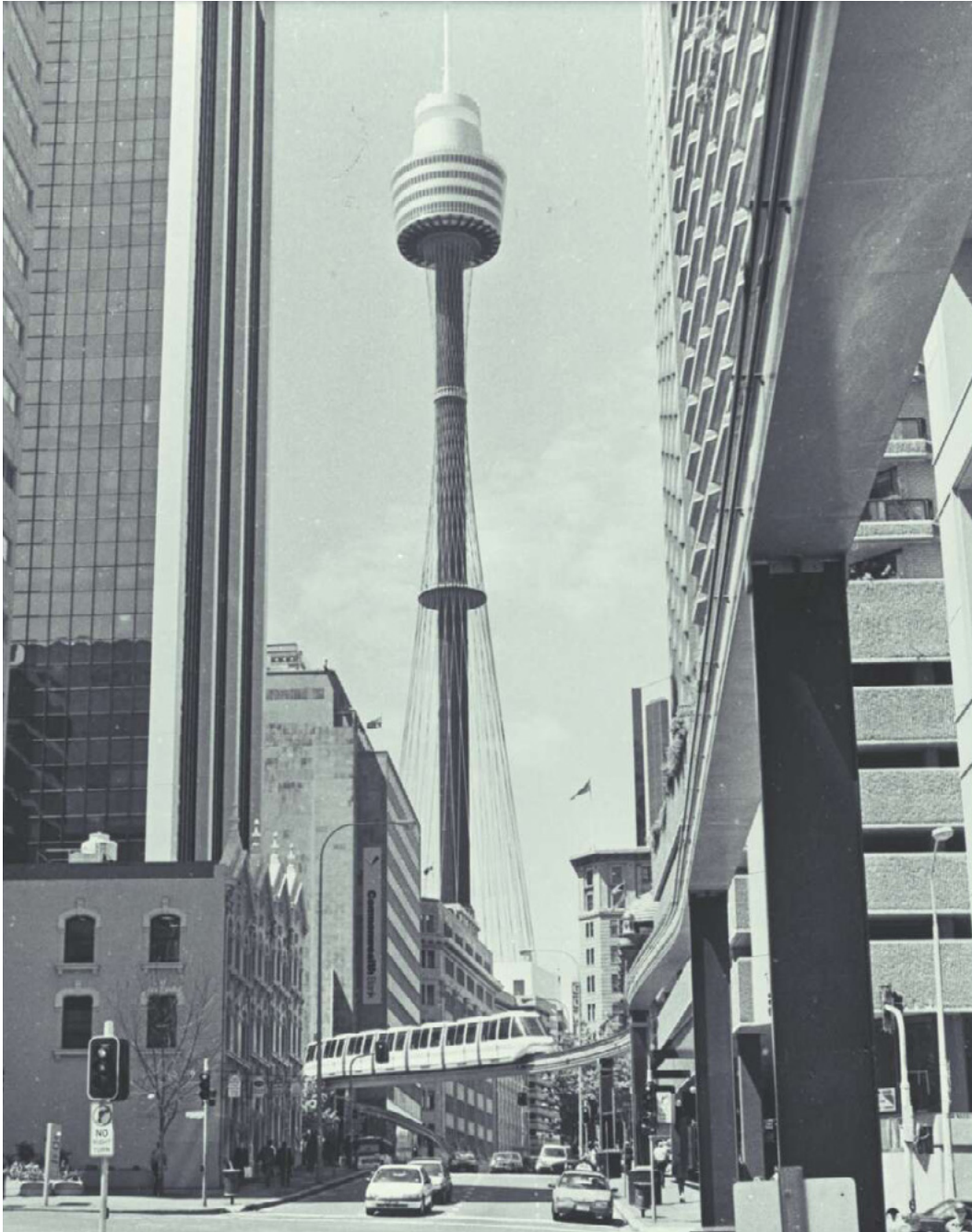
Figure 54 Centrepont Tower, Sydney, designed by Donald Crone & Associates, completed 1974
