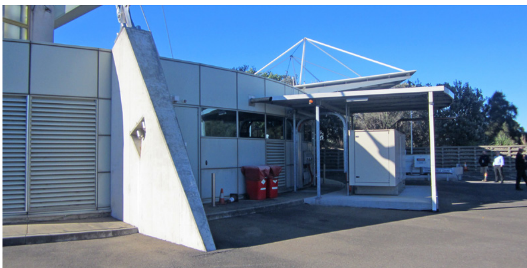
Figure 21 View of the base building from the west: the cantilevered awning outside the equipment room is visible to the rear
