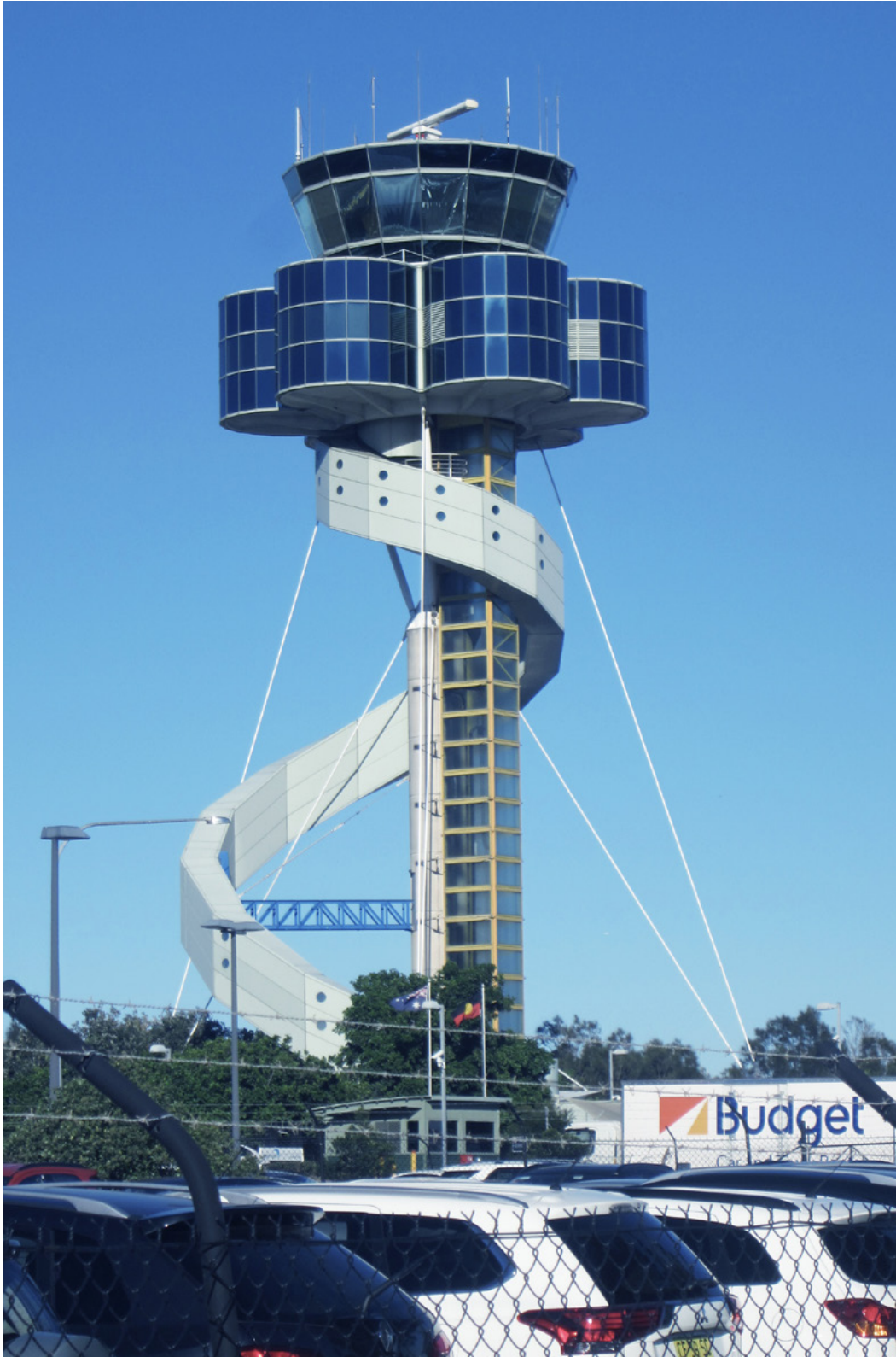
Figure 15 Sydney ATC tower no. 5, 2016, view from the east
