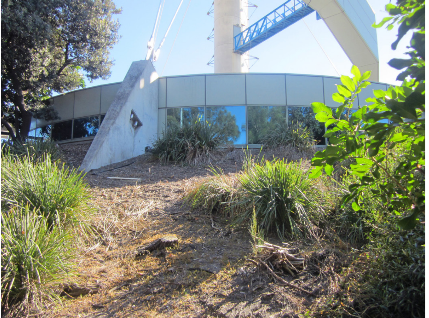
Figure 18 View of the base building from the south
