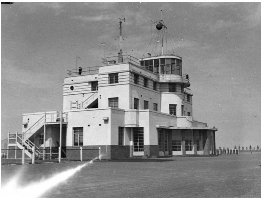
Figure 10 Sydney ATC tower no. 2, 1941
