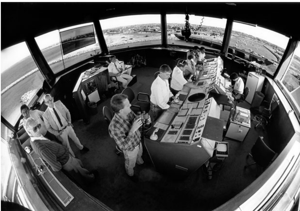
Figure 13 Inside Sydney ATC tower no. 4, 1989
