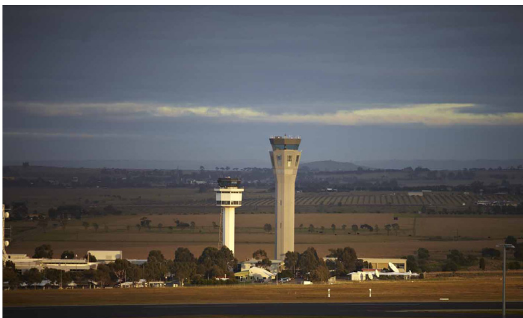
Figure 38 Melbourne ATC tower no. 1, commissioned 1969 (left) and ATC tower no. 2, 2013 (right) www.melbourneairport.com.au , accessed 5 August 2016
