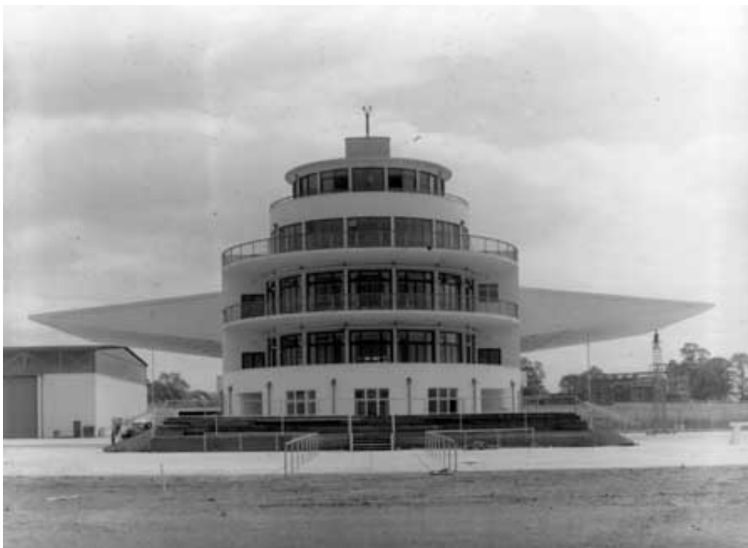
Figure 43 Integrated terminal building and control tower at Elmdon Airport, Birmingham, England, built 1939
