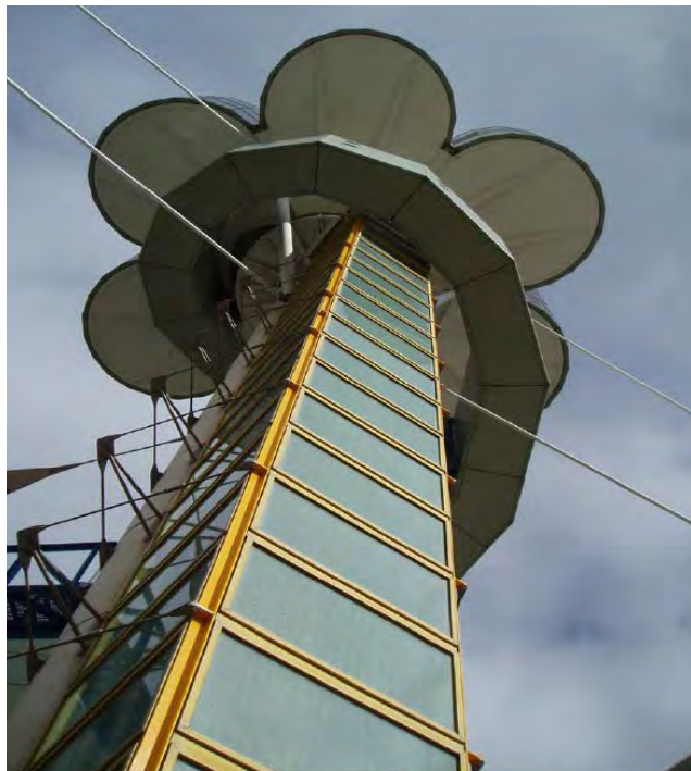
Above: View of tower illustrating significant elements
